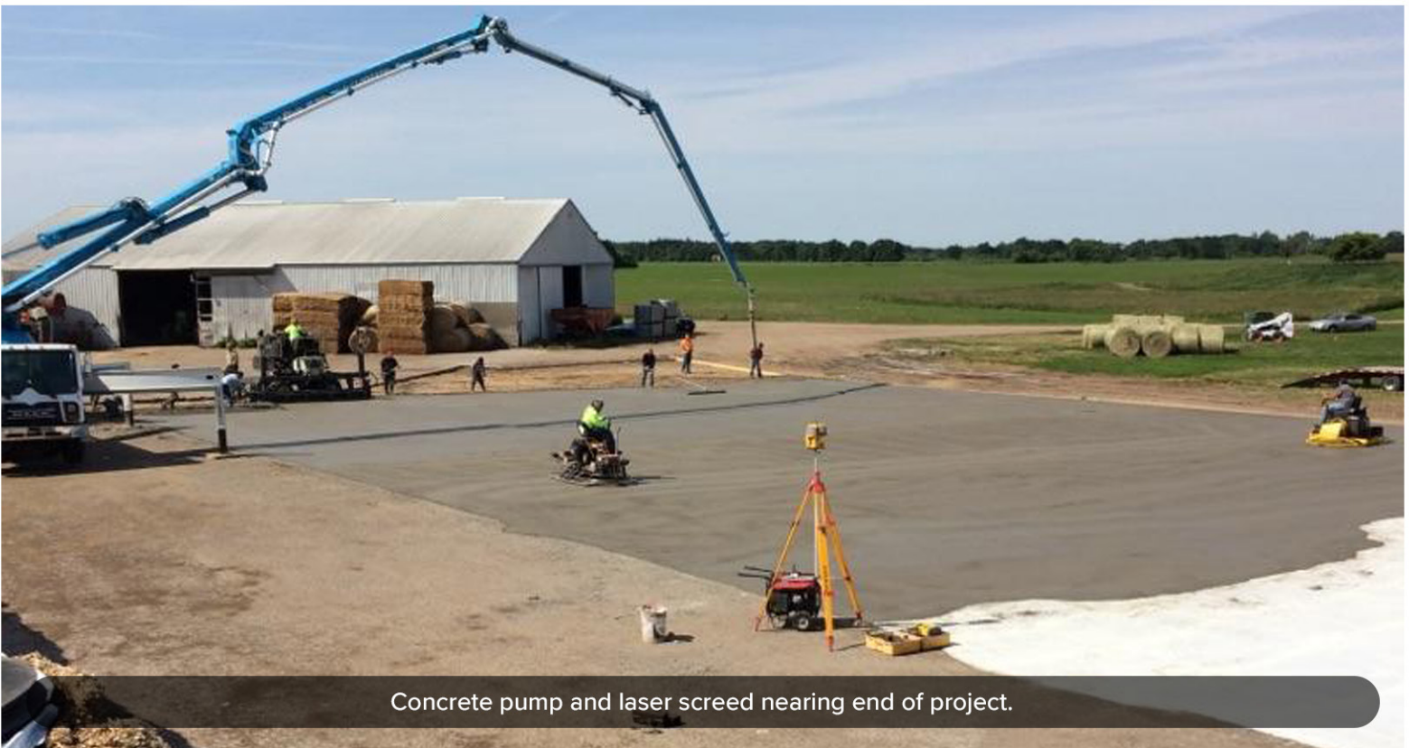
Pouring and screeding 585 yards for concrete silage slab.
